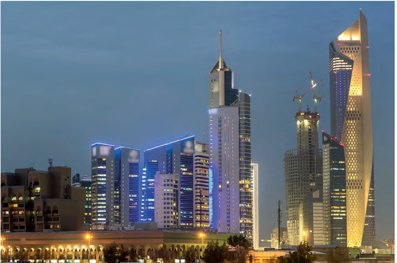
Al Hamra Tower · Kuwait
